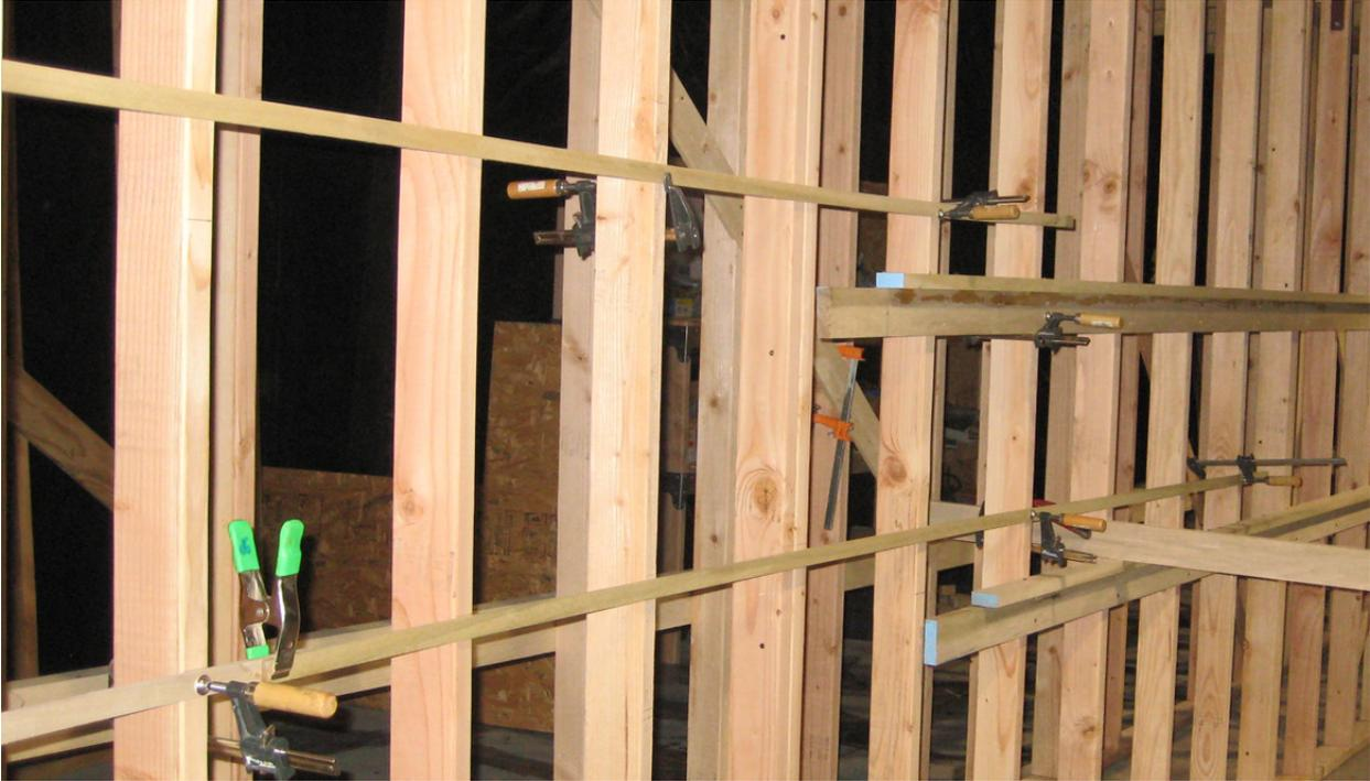
Track level strips coming into Hereford on the upper level and into Panhandle on the lower level. There will not be any L-Girders on the upper level. This one is used for study purposes only.
