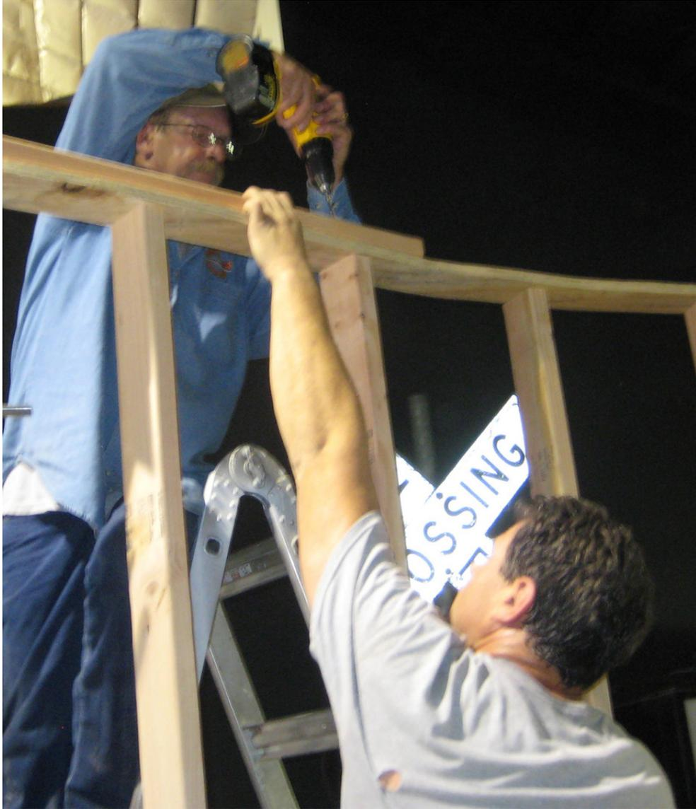
Earl Carrell and Carter Osborne are adding a second plate to the wall section. This top plate reinforces the joints between wall sections and strengthens the plates to support the roof trusses.
