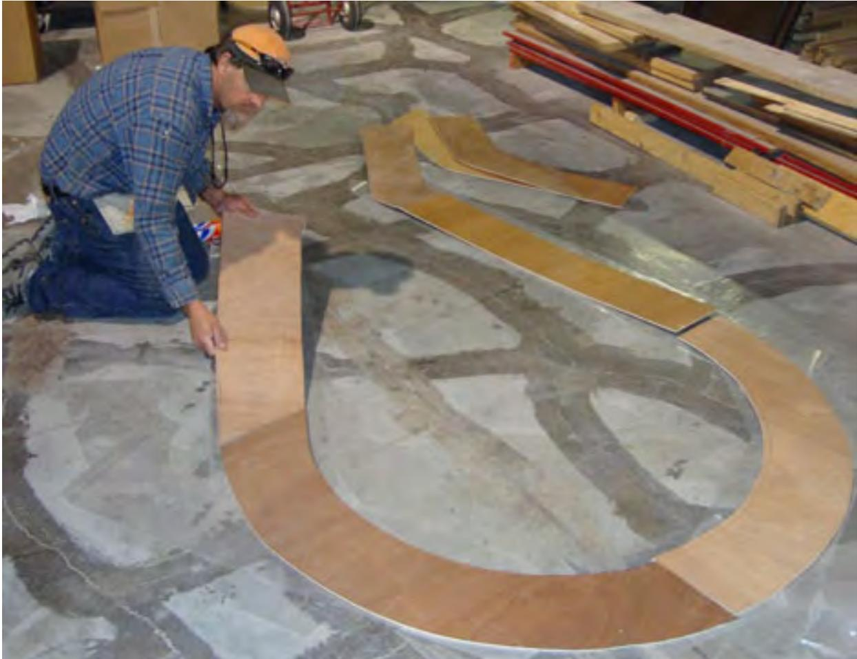
Tracy beginning work on the Canyon Wye, helix and upper level return loop for the upper staging yard. The big circular piece will be split to that the upper half can form a helix passing under itself and entering the return loop.
