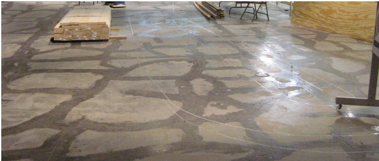
Can you see the silver lines on the floor? The inside line is the wall outline, while the outside line is the roof perimeter
