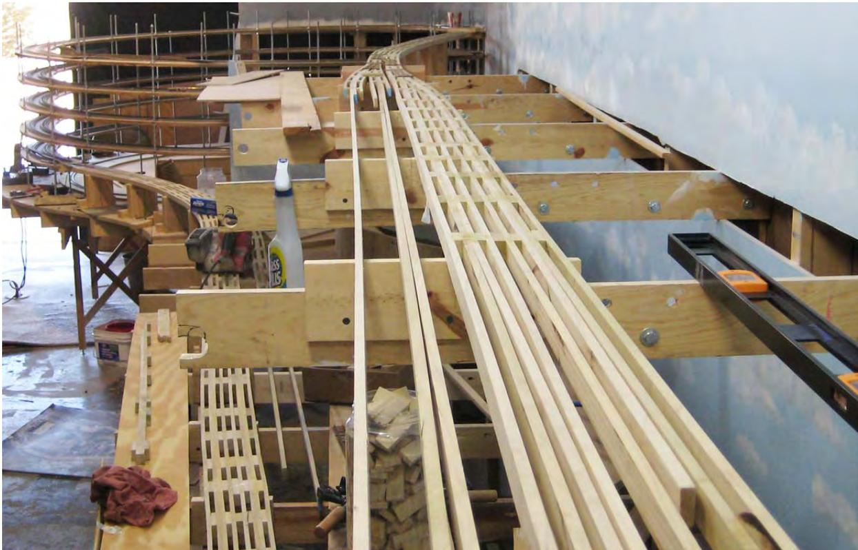
Upper level spline roadbed coming from upper level of the helix. The two lines from the helix become four lines just this side of the bridge. Two lines are almost finished while the other two lines just barely have the spine laid out.
