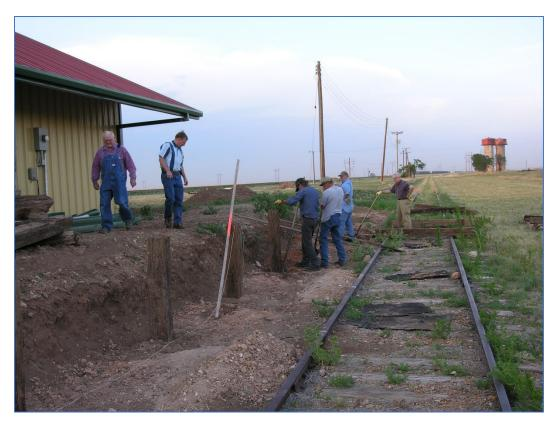
**Above**. With the building up, we needed to provide a 'loading platform' for a way to access cars in the future. A retaining wall was built in June of 2006. In both images, holes are being dug and timbers leveled and set. From left to right, Joe Sweeny, Bob Roth, Tracy Ball, Earl Carrel, Virgil Doyle, and Virgil Young. Photographer Jerry Michels. **Below**. Hard work but a comfortable spring day in the Panhandle.
