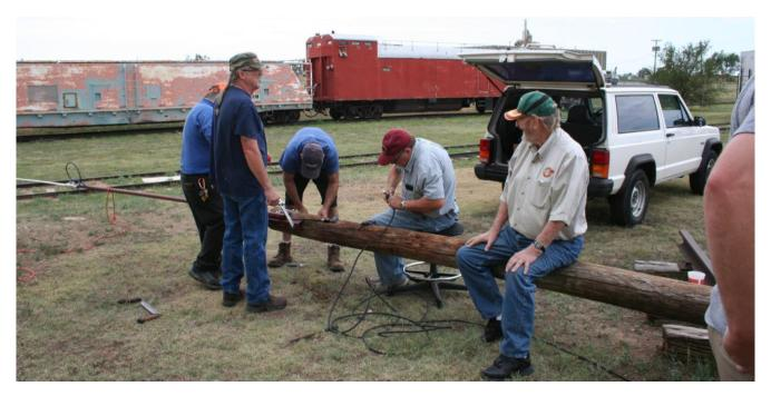
August 8, 2020: Final preparations before setting the pole with the ACTS antenna. From the left, Jimmy and Chris watching, Tracy tightening bolt securing antenna mast to the pole, Kenneth installing connector on end of cable, and Virgil holding down the top end of the pole which is balanced over the piece of railroad track.
