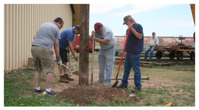
August 8, 2020: Backfilling the pole: Brian ready with next scoop of dirt while Tracy adds some water and Kenneth works on compacting the fill already in the hole; Chris waiting for signal to add his next scoop of dirt.
