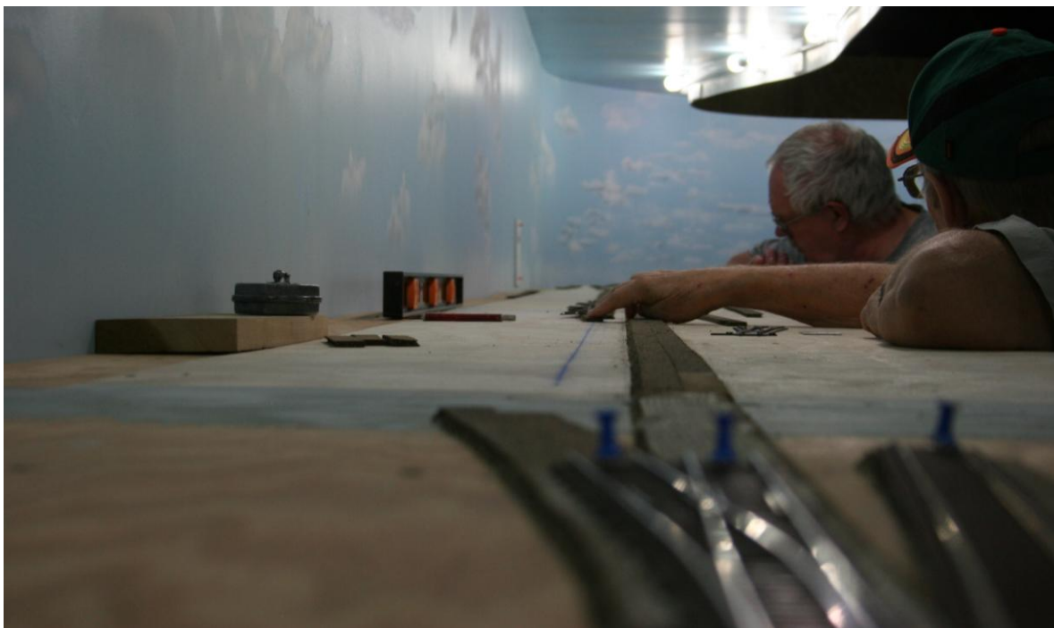
January 24, 2019: David Jusiak assisting Virgil Doyle in laying-out the location of switches on the new plywood deck at Hereford.
