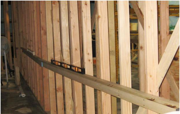
L-Girder along the inside wall of the peninsula. Sheet rock will be installed about 4 and 1/2 inches above the top of the L-Girder.
