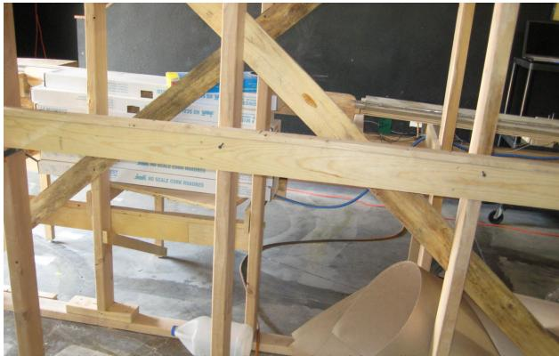
L-girder applied to wall under Umbarger location. The backdrop will be spaced just above the L-girder and will reach four feet above.
