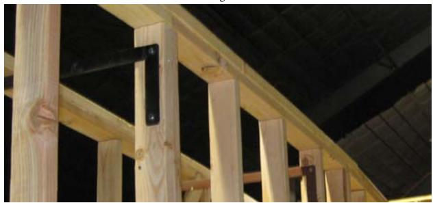
While Virgil Doyle was clamping track, Jerry Michels doubled the plates on the remaining walls. This stiffens the joints between wall sections and provides more support for the roof girders.
