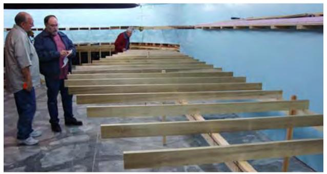
This is where it is all headed: Amarillo Junior Yard bench work temporarilly in place. There will be a narrow access aisle between the wall and the yard. The main line will run down the wall side. Our narrowest members will clear up derailments, etc. in this area.
