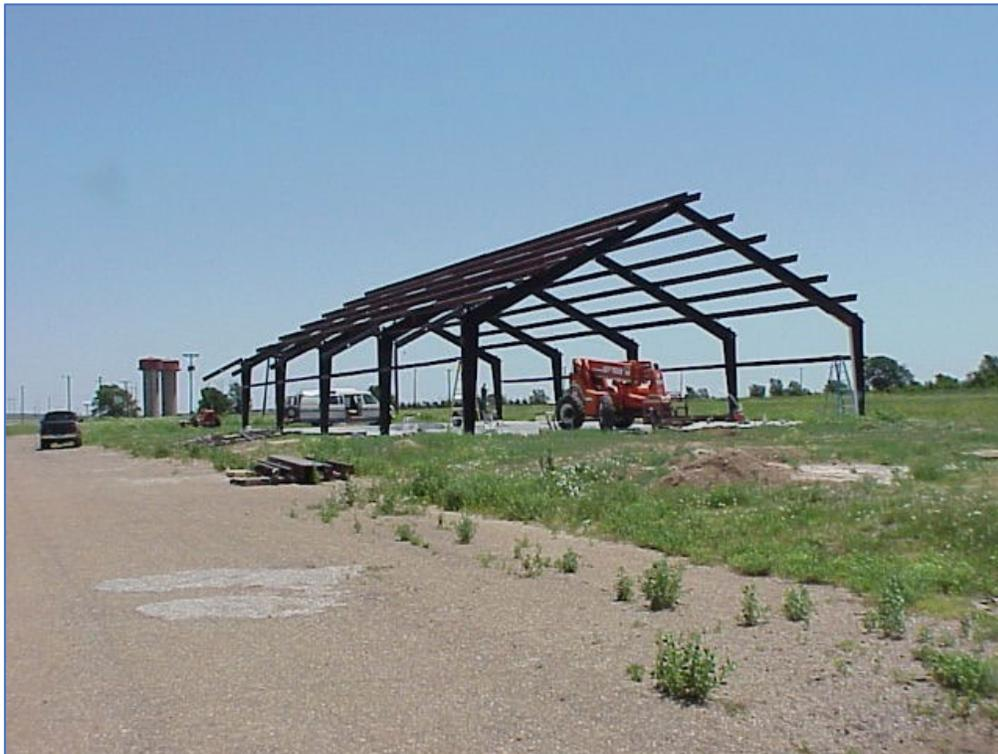
The foundation was laid, and steel went up quickly (2003-07-04). In-slab plastic coils were installed for heat. Then member Tom Jones (now enjoying Idaho) was the primary contractor and gave us a fantastic discount. As a note, the entire area is a series of east-west berms on which warehouses were built. The tracks
