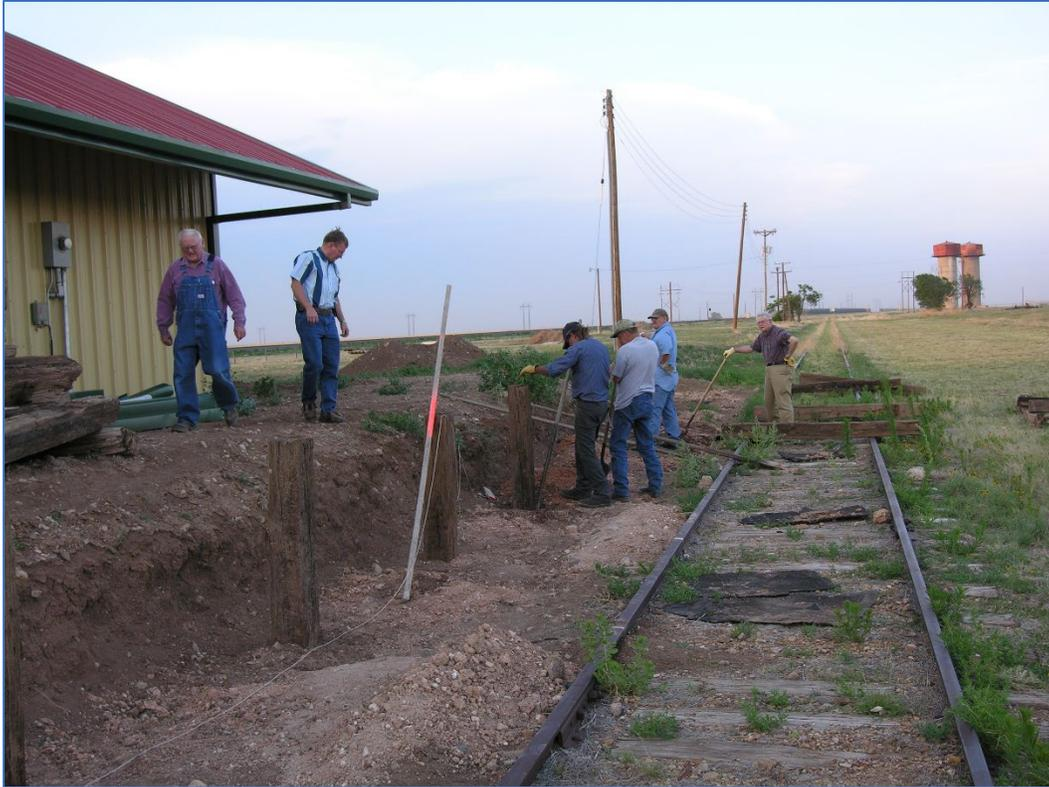
**Above.** With the building up, we needed to provide a 'loading platform' for a way to access cars in the future. A retaining wall was built in June of 2006. In both images, holes are being dug and timbers leveled and set. From left to right, Joe Sweeny, Bob Roth, Tracy Ball, Earl Carrel, Virgil Doyle, and Virgil Young. Photographer Jerry Michels. **Below.** Hard work but a comfortable spring day in the Panhandle.
