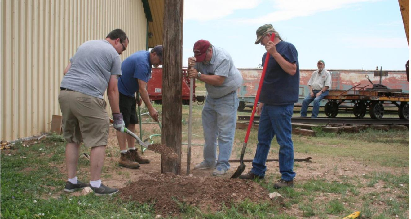
August 8, 2020: Backfilling the pole: Brian ready with next scoop of dirt while Tracy adds some water and Kenneth works on compacting the fill already in the hole; Chris waiting for signal to add his next scoop of dirt.
