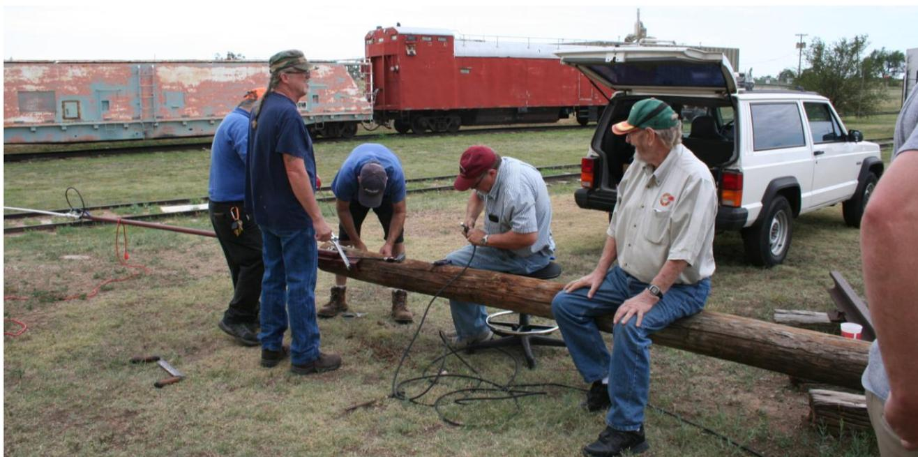
August 8, 2020: Final preparations before setting the pole with the ACTS antenna. From the left, Jimmy and Chris watching, Tracy tightening bolt securing antenna mast to the pole, Kenneth installing connector on end of cable, and Virgil holding down the top end of the pole which is balanced over the piece of railroad track.
