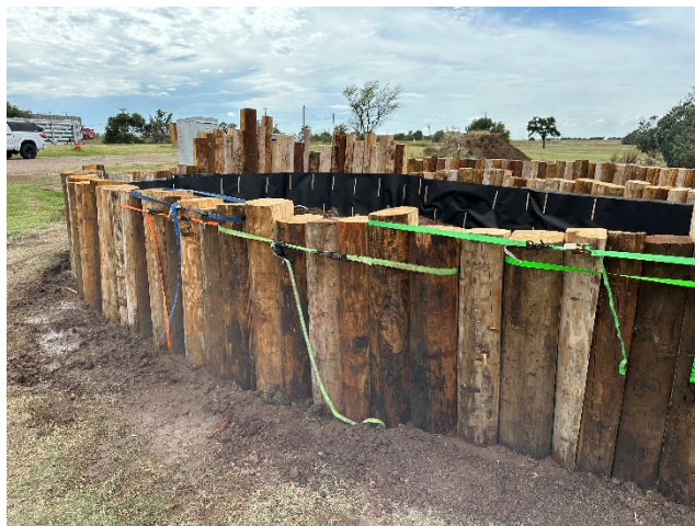
Figure 6 Exterior view of retaining wall, straps used for setting poles
