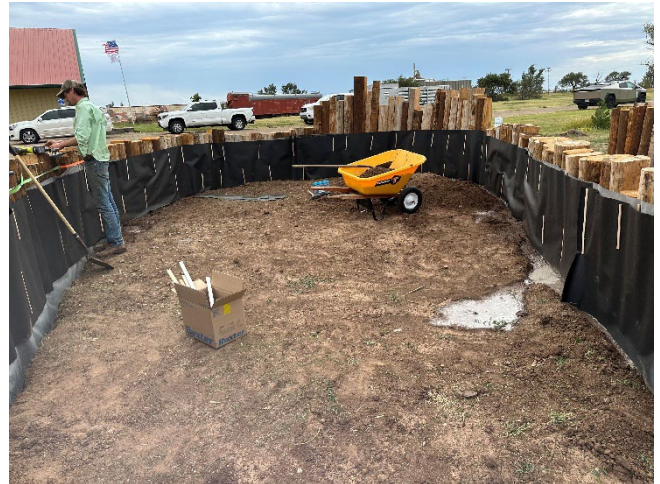
Figure 5 Interior loop of retaining wall being prepared for soil installation
