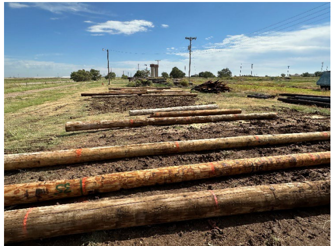
Figure 2 Utility poles staged for reduction to 6' lengths
