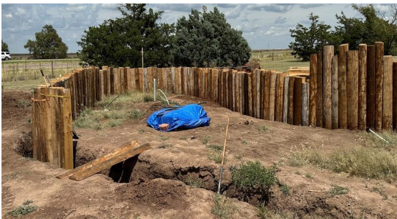
FIGURE 11 RETAINING WALL AS OF 8/18/2025
