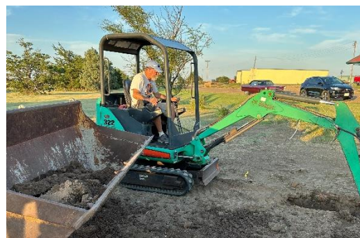
FIGURE 7 TRACY BALL DIGGING THE TRENCH FOR RETAINING WALL
