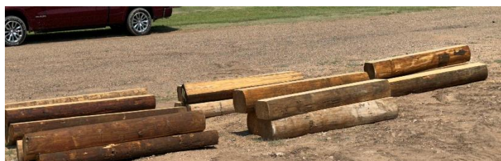
FIGURE 8 LOGS SLABBED AND READY TO SET IN TRENCH
