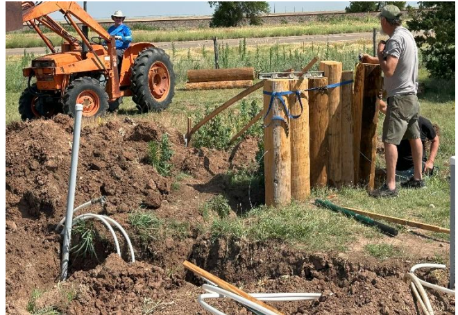
FIGURE 10 KEN WATSON AND T BALL SETTING FIRST POLES
